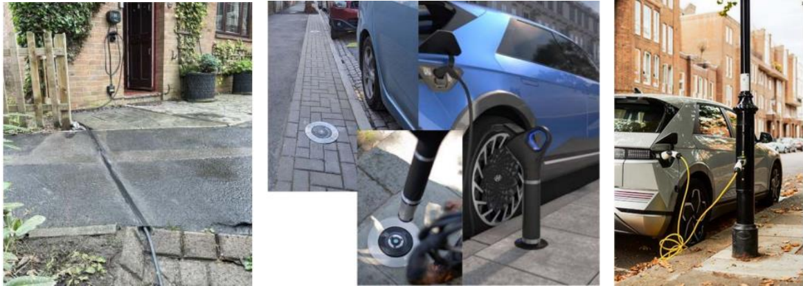
From L to R: Cable gullies; “flat and flush” charging points; lamppost charging .
